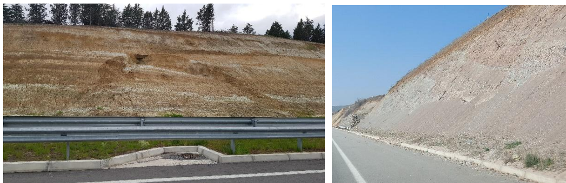
Figure 1. Examples of slope instability along the Miladinovci–Štip highway: failure of a slope section caused by berm wetting (left) and long-term erosion resulting from atmospheric effects (right).
