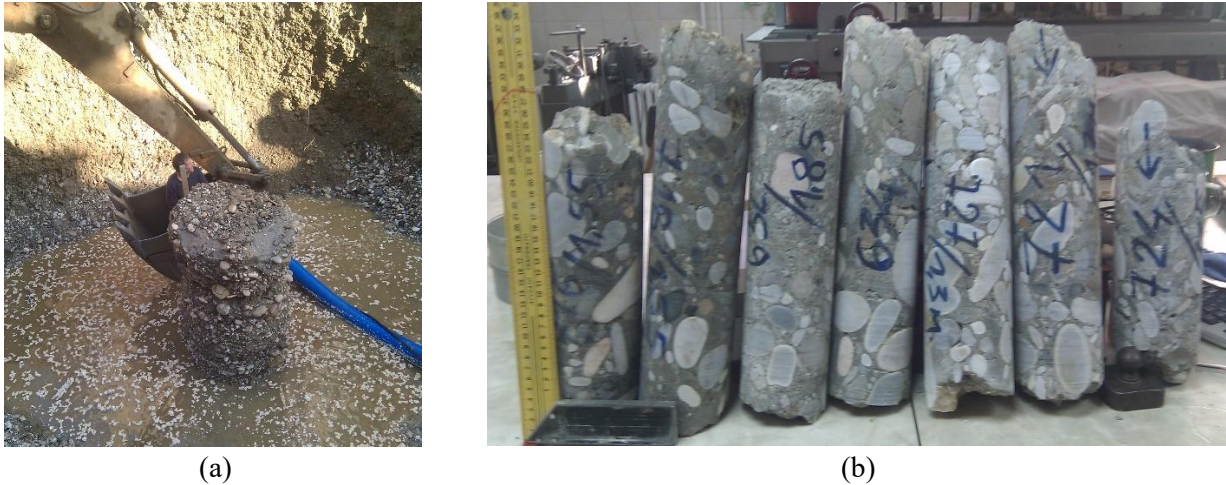
Figure 4. Field investigation – visual inspection (a) and soilcrete specimens for laboratory tests (b).
