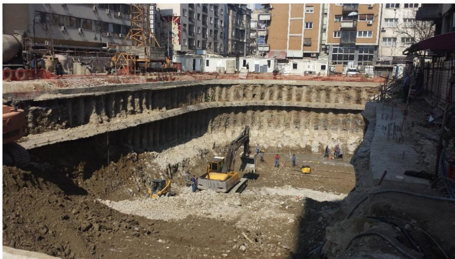
Figure 2. Excavation pit with pile retaining wall.
