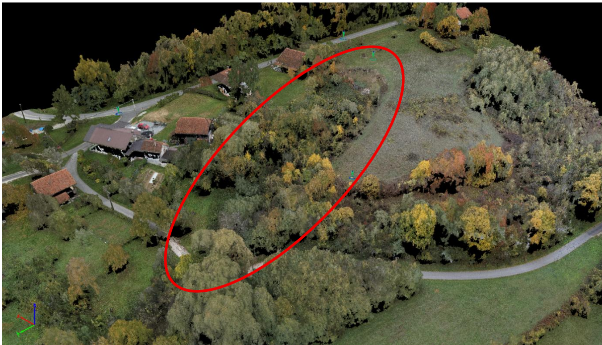
Figure 3. Photogrammetry 3D point cloud of Gornja Plemenčcina landslide marked with red line and surrounding area
