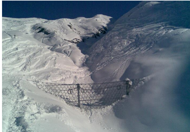
Figure 6. Barrier in Figure 5, partially covered with snow during the winter. The snow load must be considered for the final setup of the barrier. Hasliberg, Switzerland
