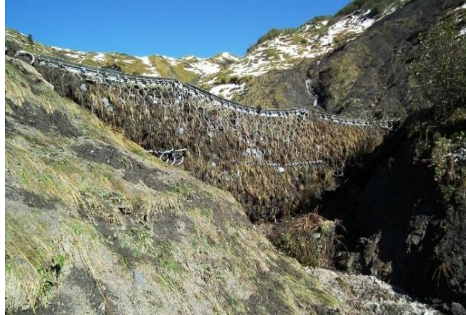
Figure 16. Eleven debris flow protection barriers, successfully filled in Hasliberg, Switzerland
