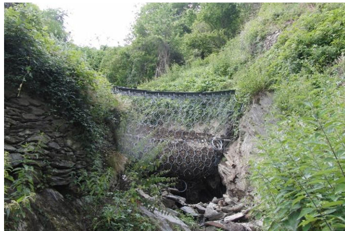
Figure 13. Partially filled debris flow barrier over the German railway near Koblenz
