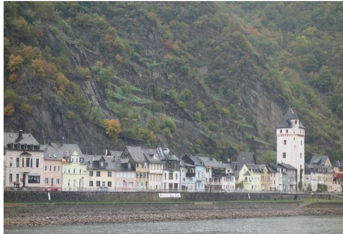
Figure 12. Almost invisible flexible barrier near Koblenz along the Rhine River above a UNESCO World Heritage village
