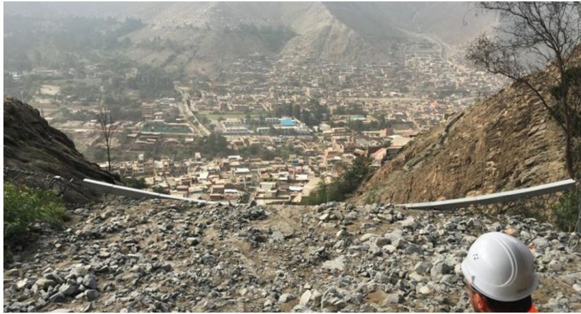
Figure 19. VX barrier successfully protecting a huge population center downstream, Chosica Peru
