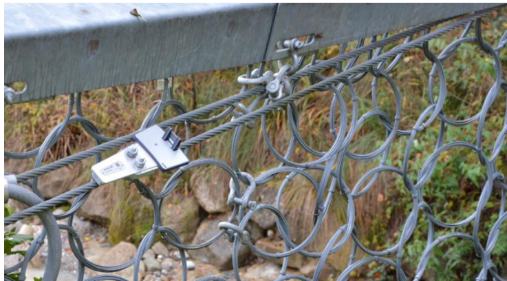
Figure 26. State-of-the-art Sensor Guard placed in a flexible barrier against debris flows
