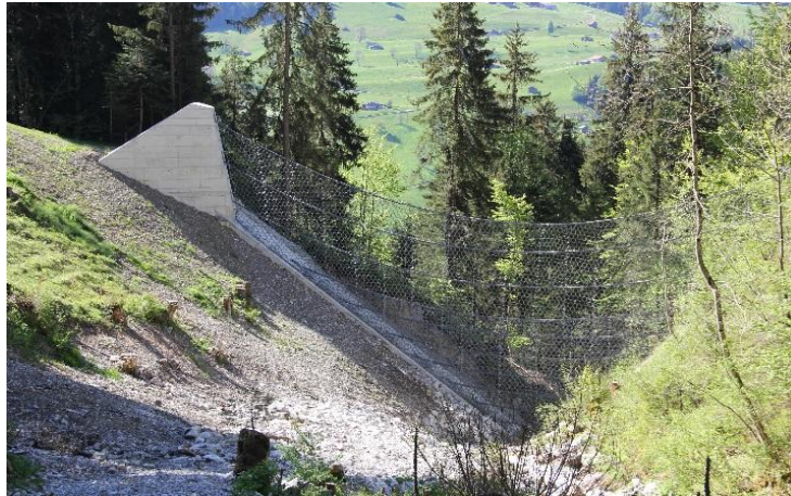
Figure 24. Special barrier solution in Hüpach, Switzerland
